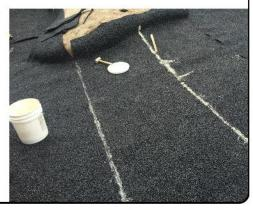
Place the edges of the pads under the turf that was lifted up in step 2. Cut to size and shape as needed. Replace turf over pad edges.
