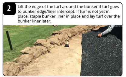
Starting from the middle of the bunker, unroll the pads and lay them so the edges touch but do not overlap. If necessary, cut pads to fit in shorter runs or to lay end to end for longer runs. Staple and / or glue ends together.
